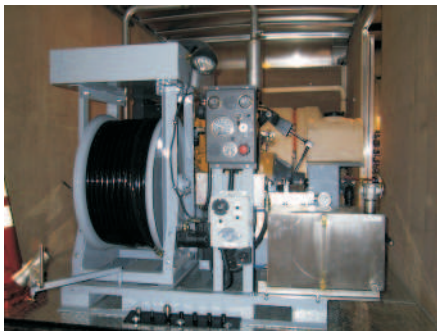
Skid Mounted Van Installation
