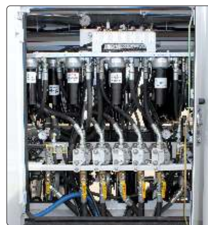
New design improves serviceability on the high pressure filters
